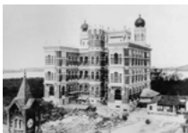
Moorish Pavilion under construction, 1907 Fonds Oswaldo Cruz Institute.
