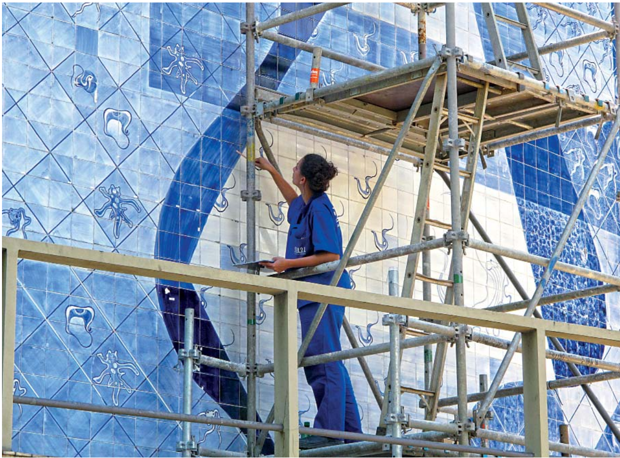
36 – Mapeamentos de danos no painel de azulejos – Surveying of the damage to the tile mural
