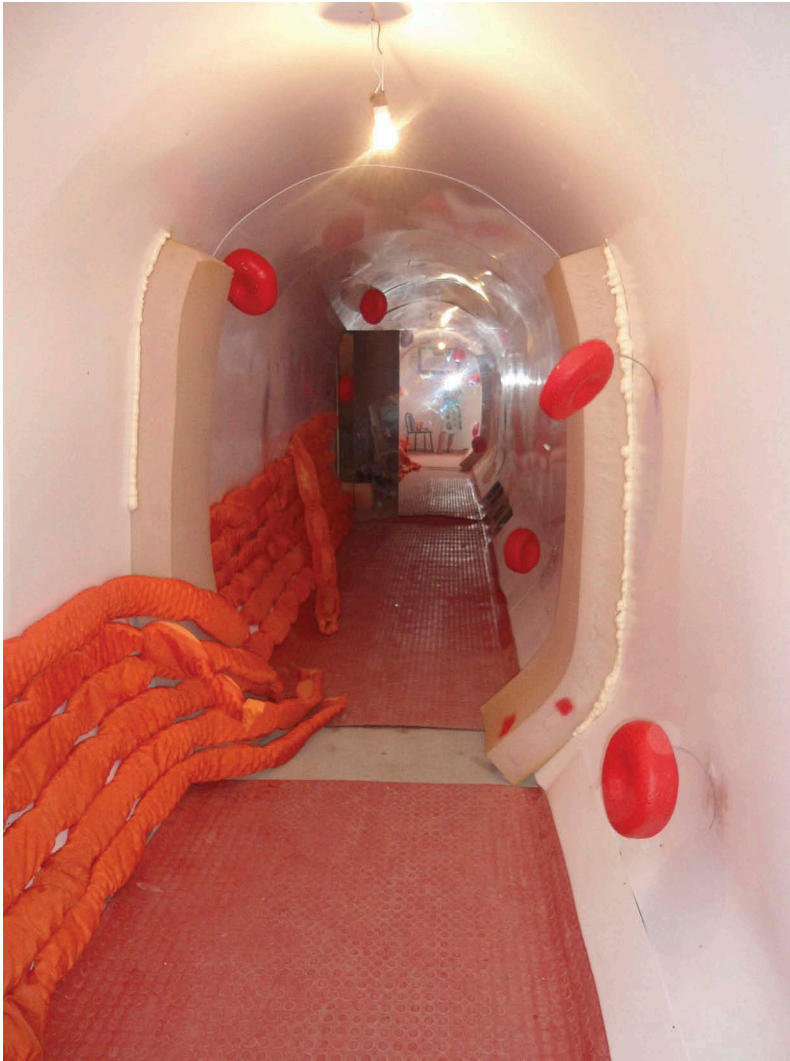
Figure 10. Phase of construction of the 'Giant Artery' using polystyrene plates.
