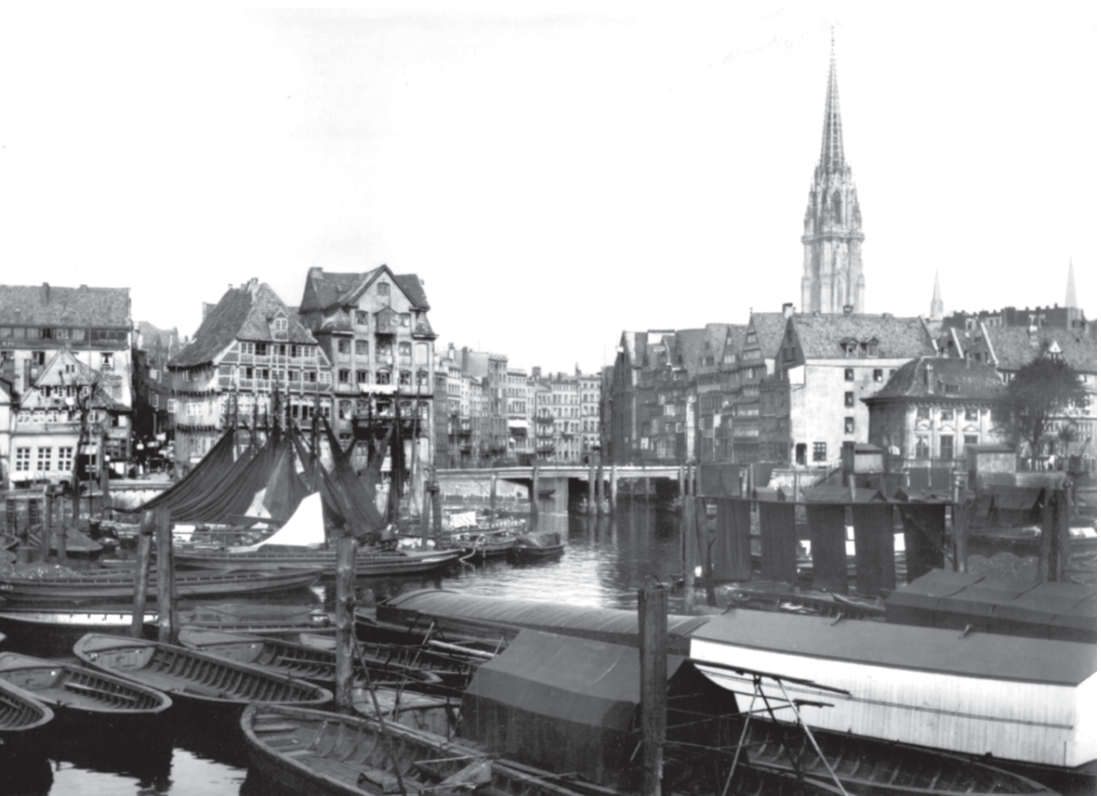
Hohe Brücke (High Bridge) seen from Kehrwieher, in Hamburg, Germany. Photo by G. Koppmann & Co., September 1884.
