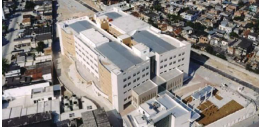
Figura 16 – Hospital Municipal Ronaldo Gazolla – "Hospital de Acari".
