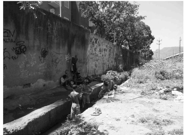
Fig. 4. Public water pipe where homeless crack users bathe, wash their clothes and do their personal hygiene.
