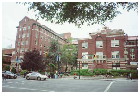
Figura 98: Fachada frontal – Prédio Burrard Building
