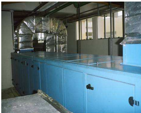
Figura 82: Fan-coil
