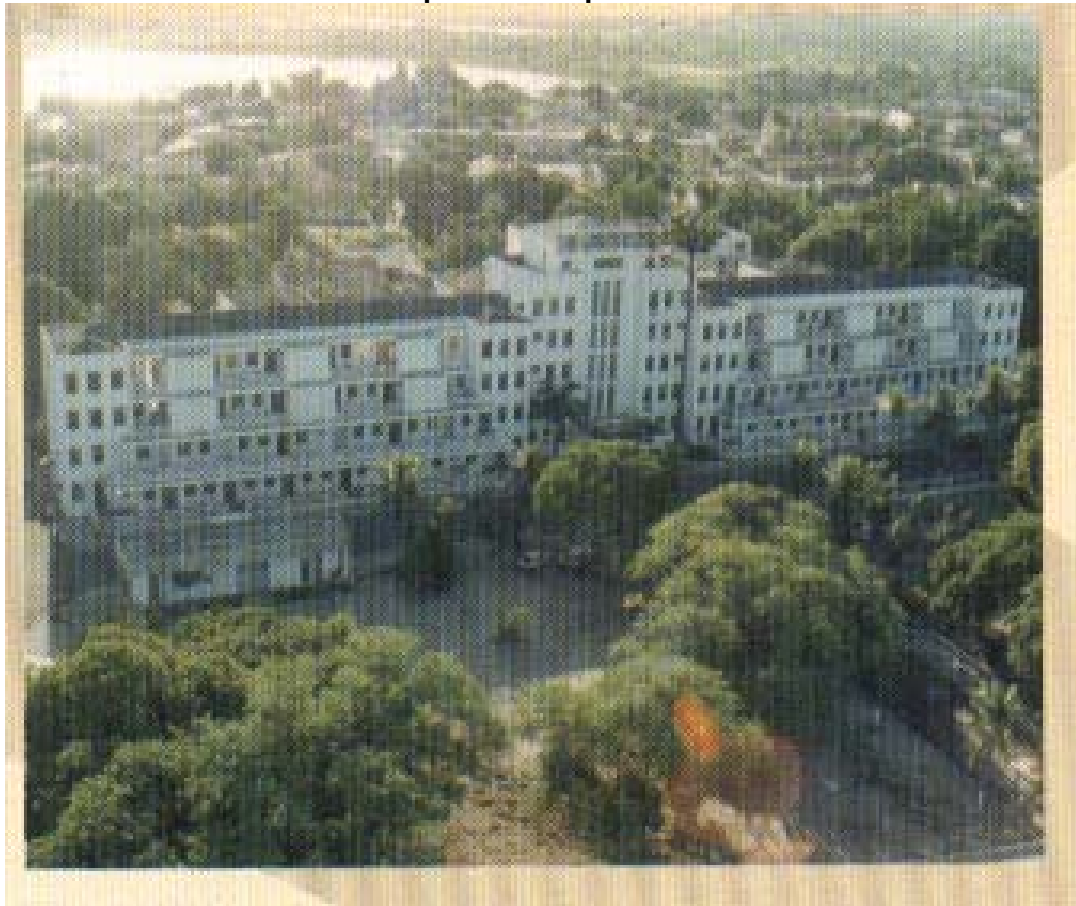
FIGURA 3.21 – Hospital Municipal de Maracanaú – 1950
