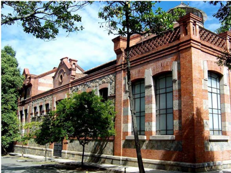
Figure 3. Stable Building. Photo: Celeste Souza.
